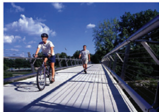
Walking and Cycling Structure, London, Ontario
