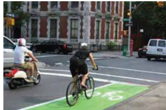
Bright Demarcation at Intersections Enhance the Concept of Crossing the Bike Lane to Vehicles and Increase Awareness
