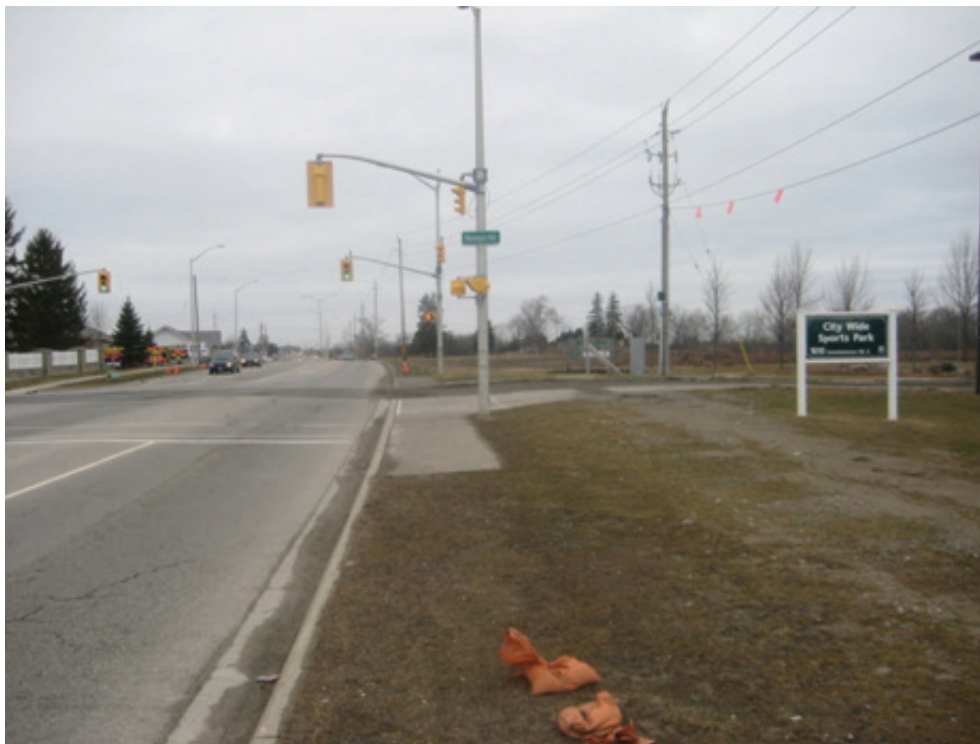
Need to Extend Sidewalk on Northeast Quadrant
