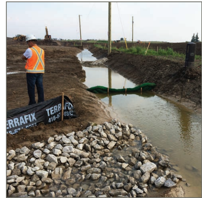
Example of erosion control measures
