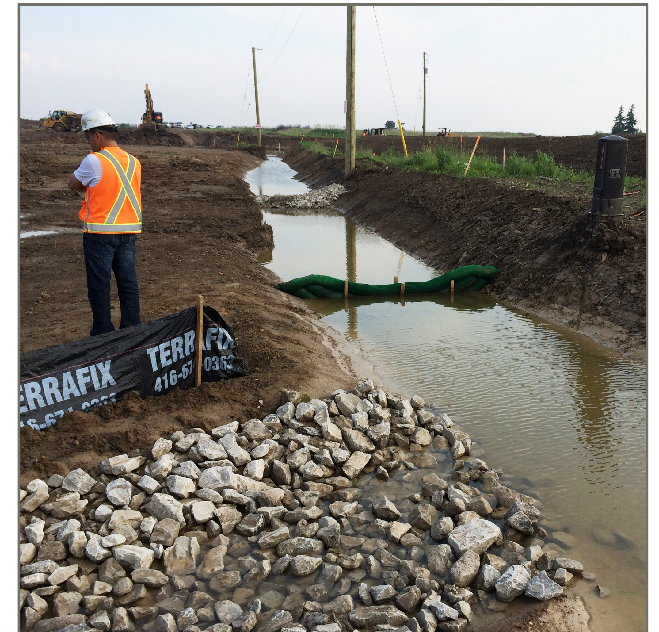
Example of erosion control measures
